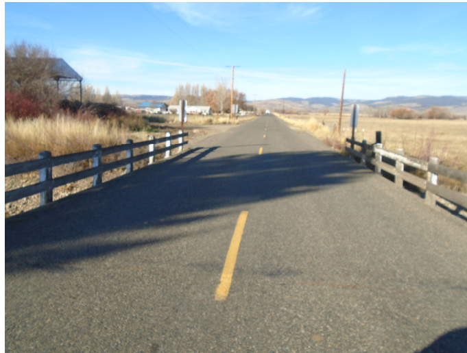
Cooke Canyon Rd looking north
